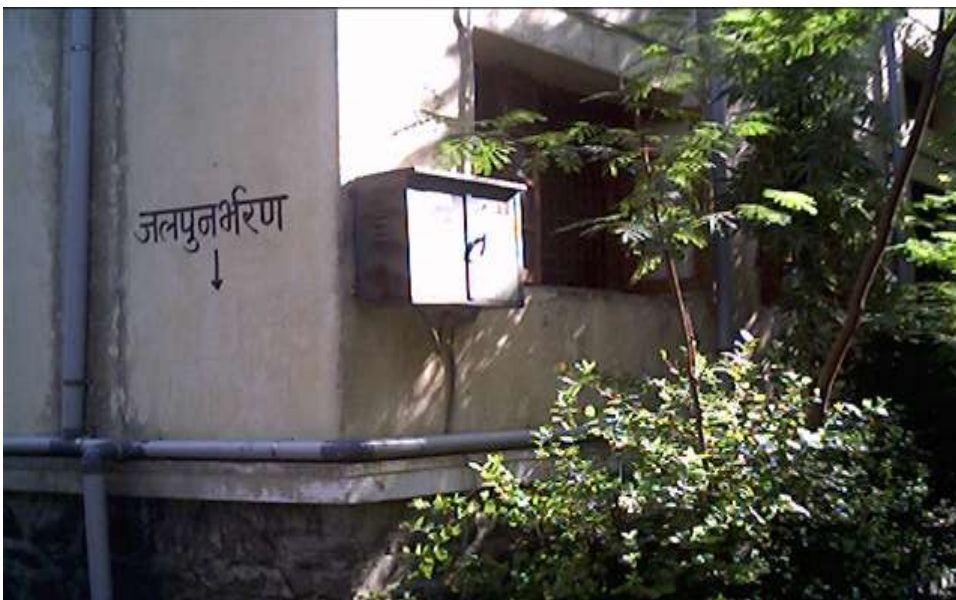
Partial view of roof water harvesting building along with vertical and horizontal PVC pipes collecting the water and control panel board for submersible in the bore well
